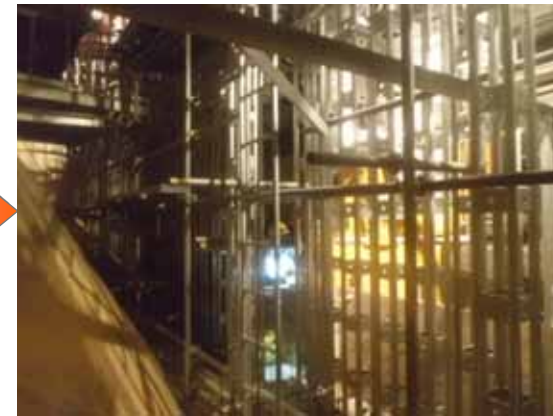
After installation of steel support pillars (June 20)
