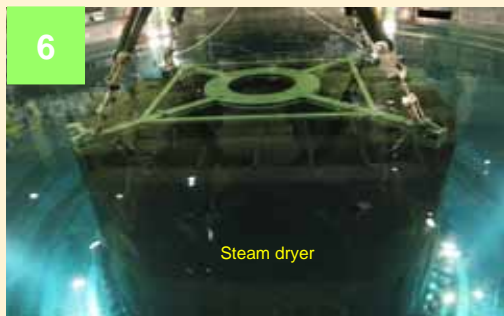
Steam dryer removal (Photo taken on September 19, 2012)
