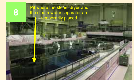
After the reactor was opened (Photo taken on September 22, 2012)
