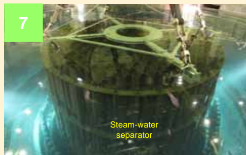
Steam-water separator removal (Photo taken on September 21, 2012)
