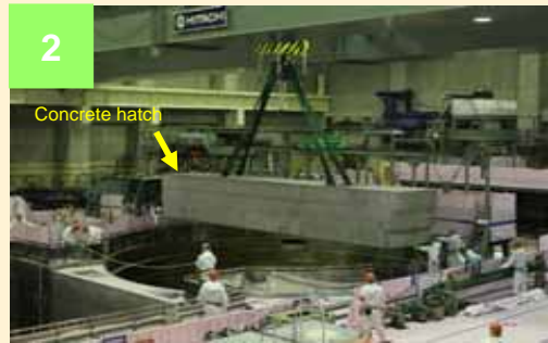
Concrete hatch removal (Photo taken on September 10, 2012)
