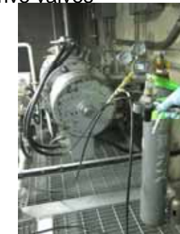
Installing a back up nitrogen gas cylinder to drive valves (Unit 3)
