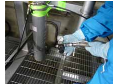
Installing a back up nitrogen gas cylinder to drive valves (Unit 3)
