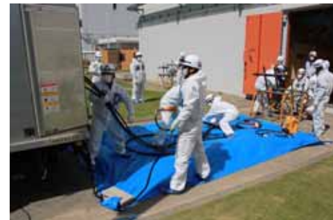
Deploying a power-supply car to the reactor building (Unit 1) Connecting power cables (Unit 1)
