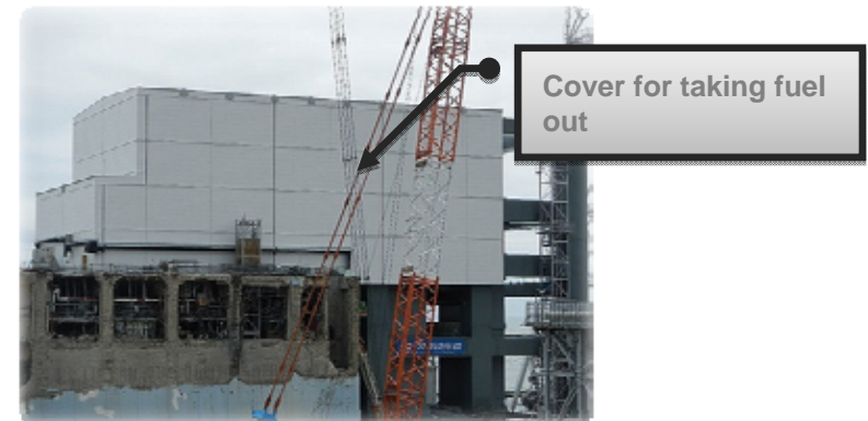
Reactor 4 with external walls and ceiling panels installed
